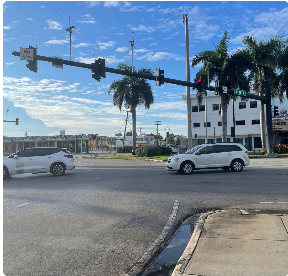
Existing traffic signal mast arm assemblies and pedestrian post mounted signals.
