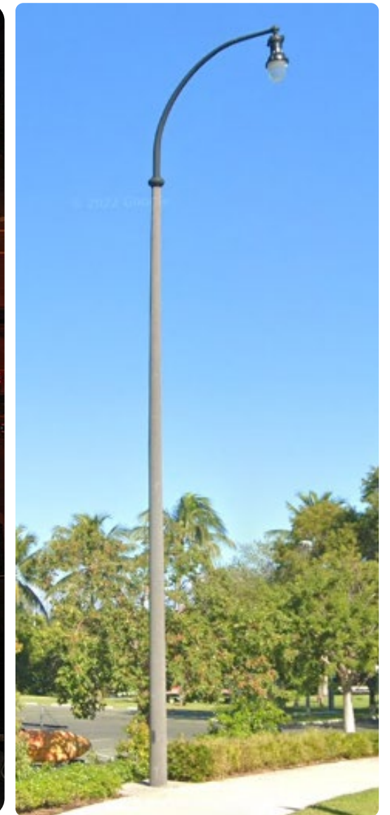
Existing decorative lighting to the east.
