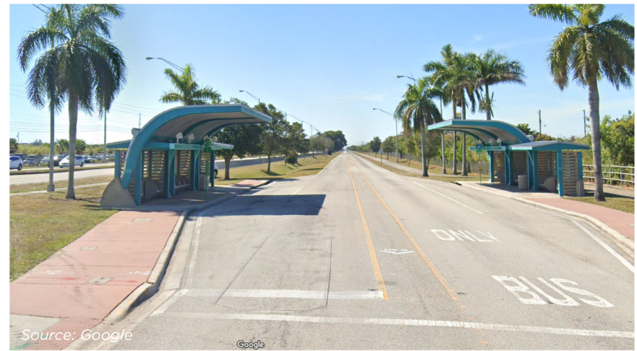
Figure 4.4.5 | Busway in Miami, Florida.
