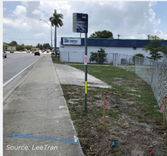
Figure 3.5.8 | Bus stop after fence was moved back.
