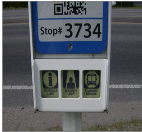
Figure 3.10.3 | Details of a solar-powered bus stop signpost with bus flagging capability and security lighting, Pinellas County, Florida.
