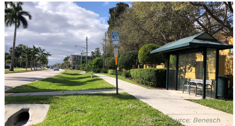
Figure 3.1.8 | B&A area connected to sidewalk and bus stop shelter along a flush shoulder roadway.
