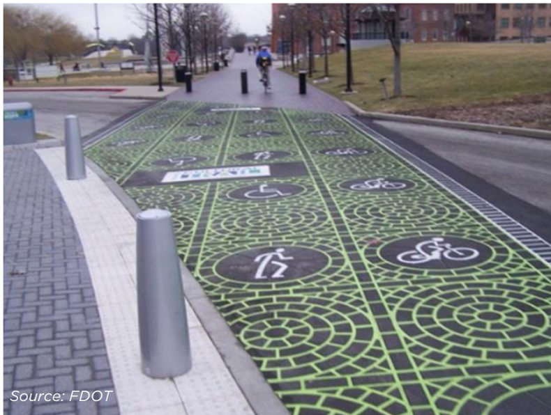
Figure 3.10.5 | Multi-use trail crossing in Indianapolis, Indiana, with decorative inlaid thermoplastic design.
