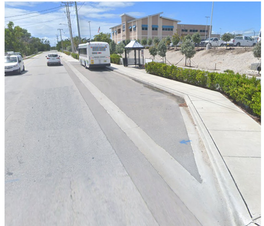
Figure 4.5.9 | Asphalt bus bay in Key West, Florida.
