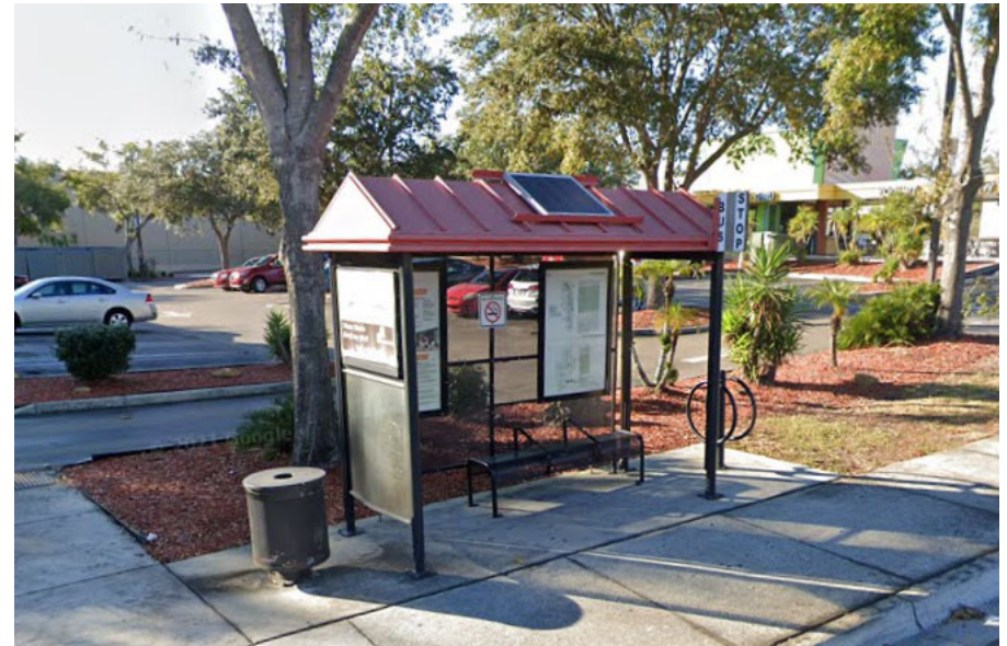
Figure 3.10.2 | Bus shelter with a solar panel, Polk County, Florida.
