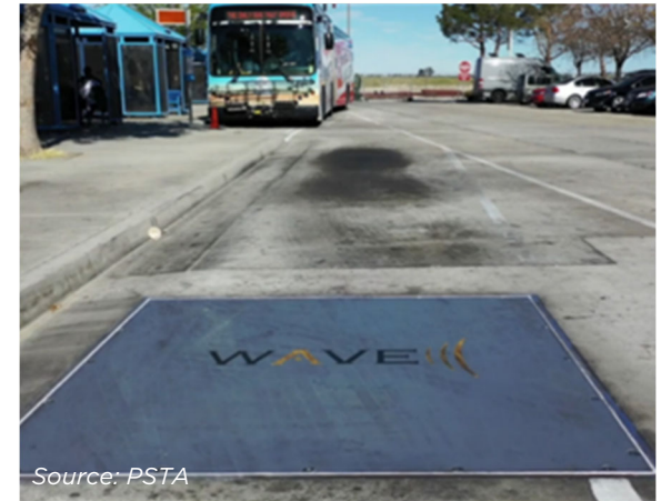
Figure 3.9.3 | Inductive bus charging station in St. Petersburg, Florida.
