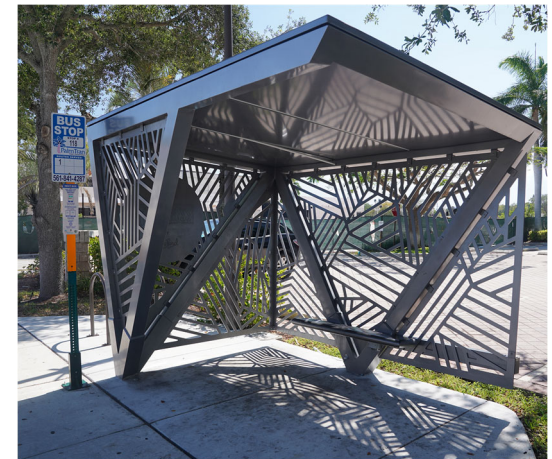
Figure 3.9.6 | Innovative bus shelter design in Palm Beach County, Florida.
