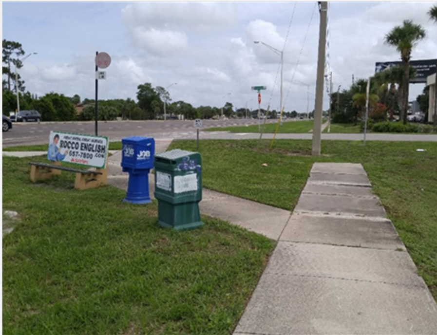
Figure 3.3.4 | Before accessibility improvements.
