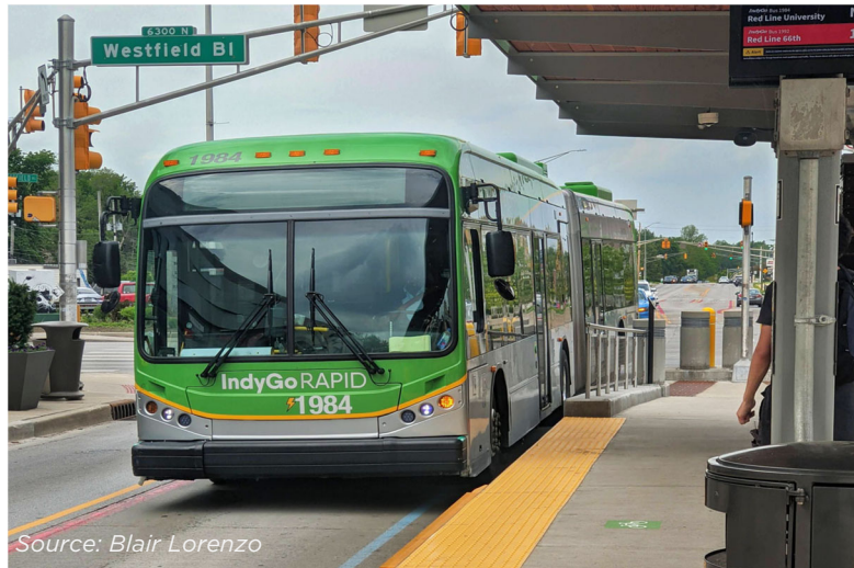
Figure 5.3.1 | Example of a median platform BRT station with near-level boarding.
