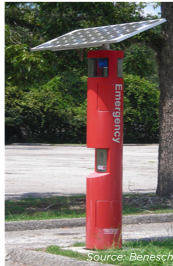
Figure 3.8.11 | Solar-powered emergency call box.
