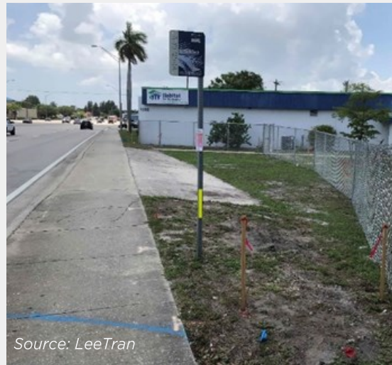
Figure 3.5.8 | Bus stop after fence was moved back.
