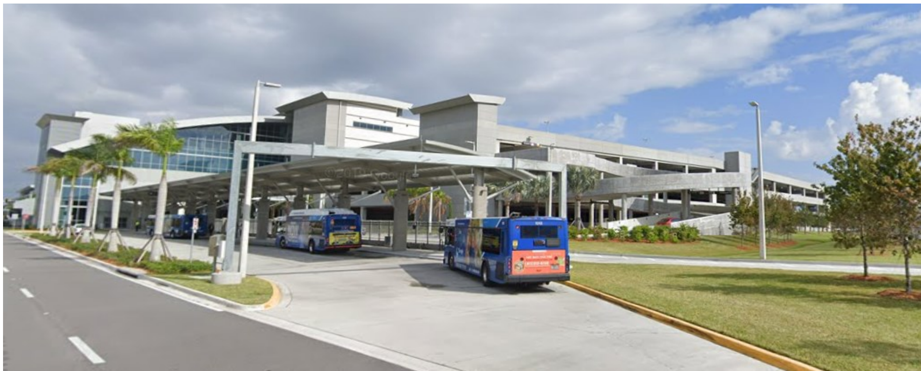
Figure D.7.1 | Bus-air intermodal facility in Tampa, Florida.
