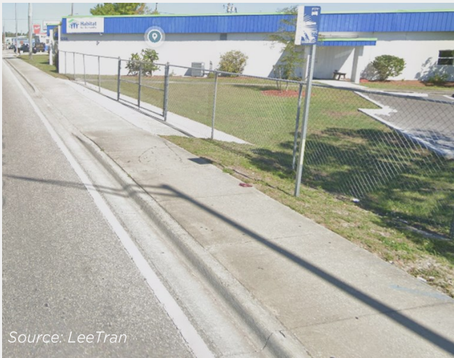
Figure 3.5.7 | Bus stop with fence limiting waiting space.
