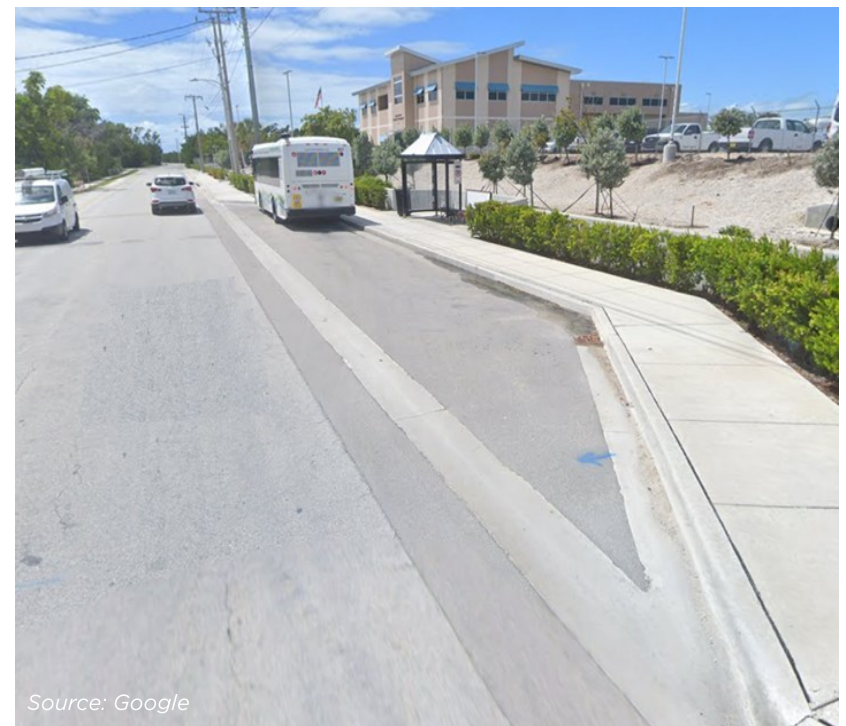
Figure 4.5.9 | Asphalt bus bay in Key West, Florida.
