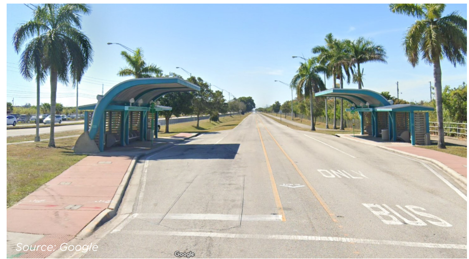
Figure 4.4.5 | Busway in Miami, Florida.
