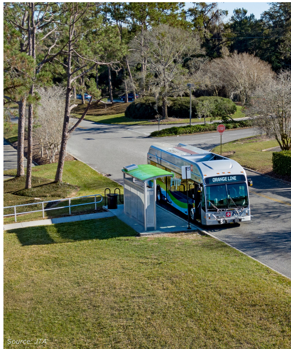
Figure 4.3.1 | On-lane bus stop in Jacksonville, Florida.
