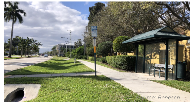
Figure 3.1.8 | B&A area connected to sidewalk and bus stop shelter along a flush shoulder roadway.
