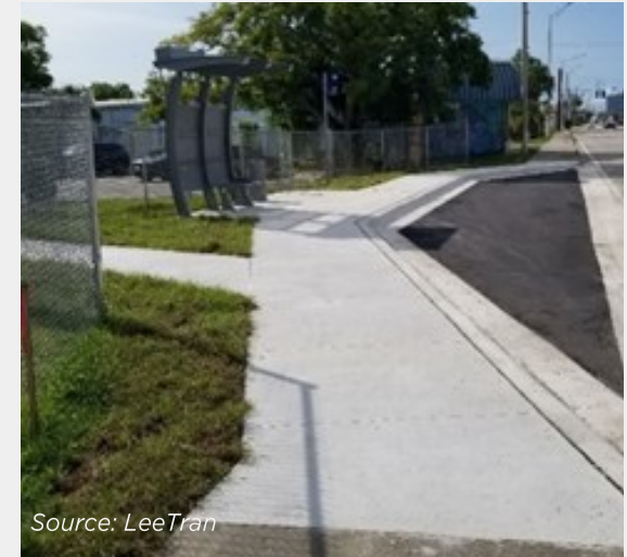
Figure 3.5.9 | Completed bus stop with bus bay and shelter.
