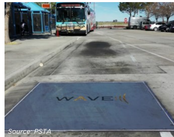
Figure 3.9.3 | Inductive bus charging station in St. Petersburg, Florida.
