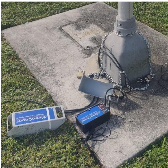
Bike tube counter installation
