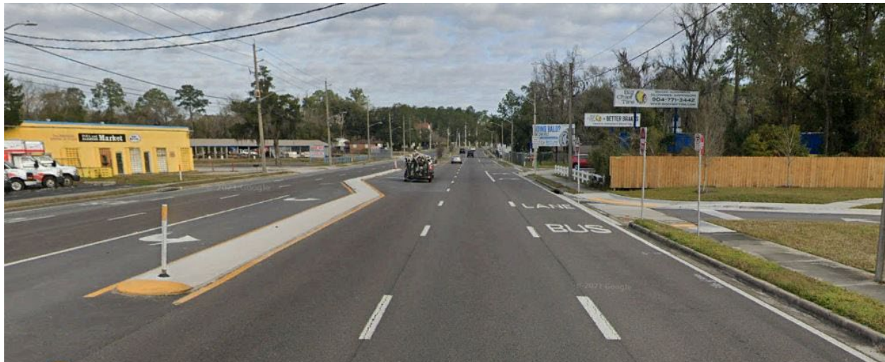
Figure 20: Blanding Boulevard Bus Only Lanes in Jacksonville, FL (Photo: Google Earth)
