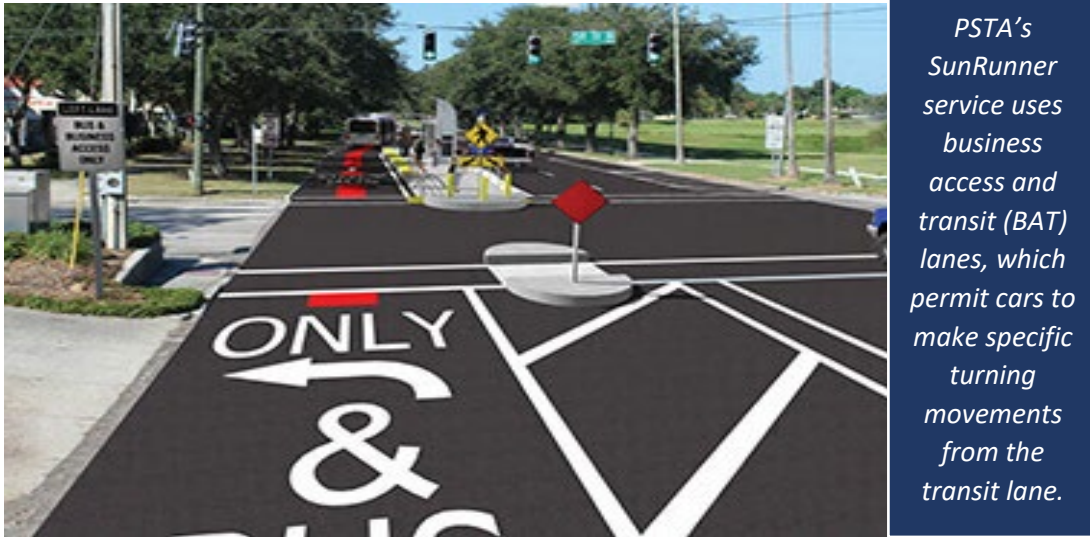
Figure 7: Pinellas Suncoast Transit Authority’s SunRunner BRT Uses Special Use Transit Lanes (Photo: PSTA)
