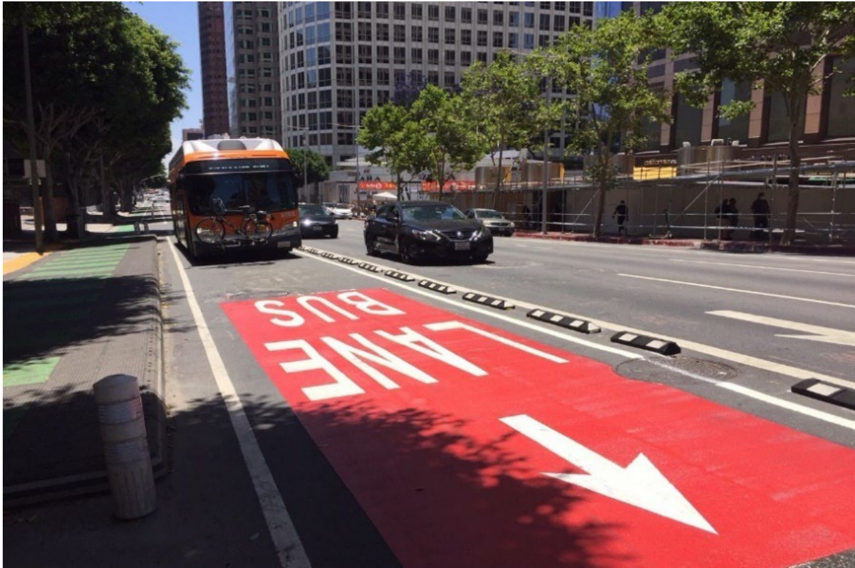
Figure 8: Red-Painted or Barrier-Separated Transit Lanes Distinguishes Them on the Roadway (Photo: Streetsblog L.A. )
