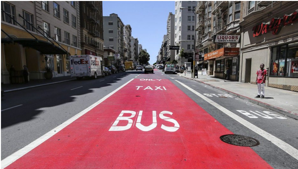
Figure 2: Example of a Special Use Lane for Buses and Taxis in San Francisco (Photo: SFMTA )
