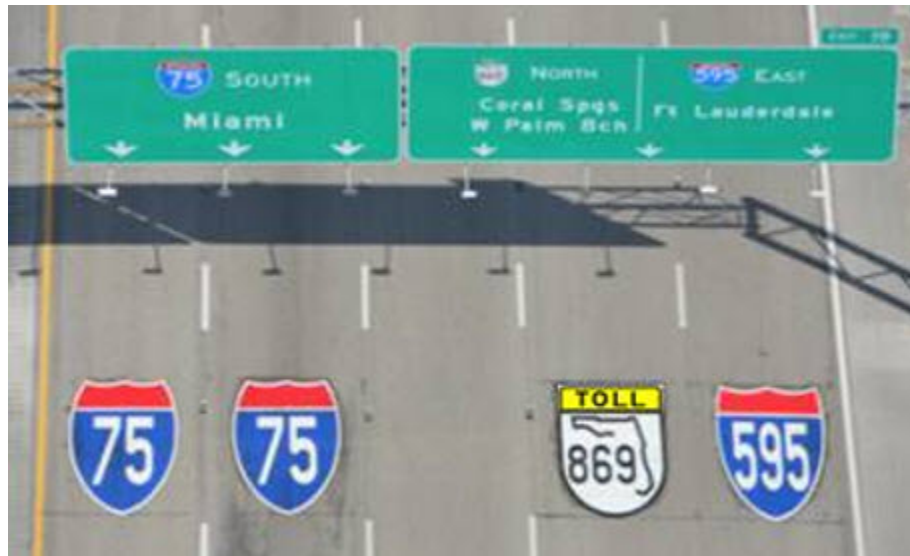
Figure 4.2-3. Route Shield Pavement Markings
