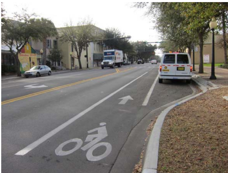
Figure 4.2-2. Pavement Symbol and Arrow Markings
