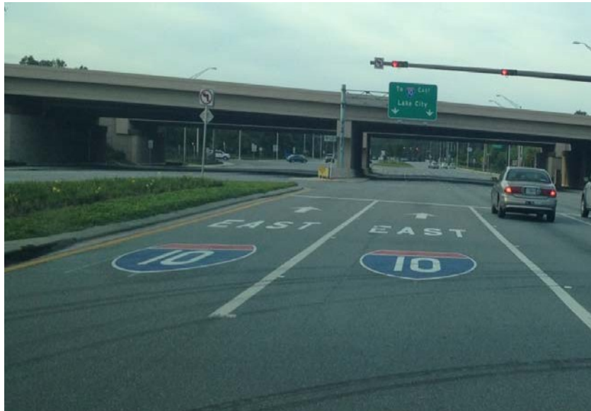
Figure 4.2-7. Pavement Markings for Wrong Way Treatment
