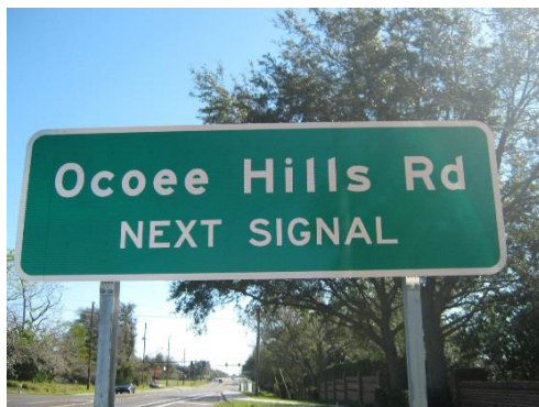
Figure 2.37-1. Advance Street Name Sign at Signalized Locations
