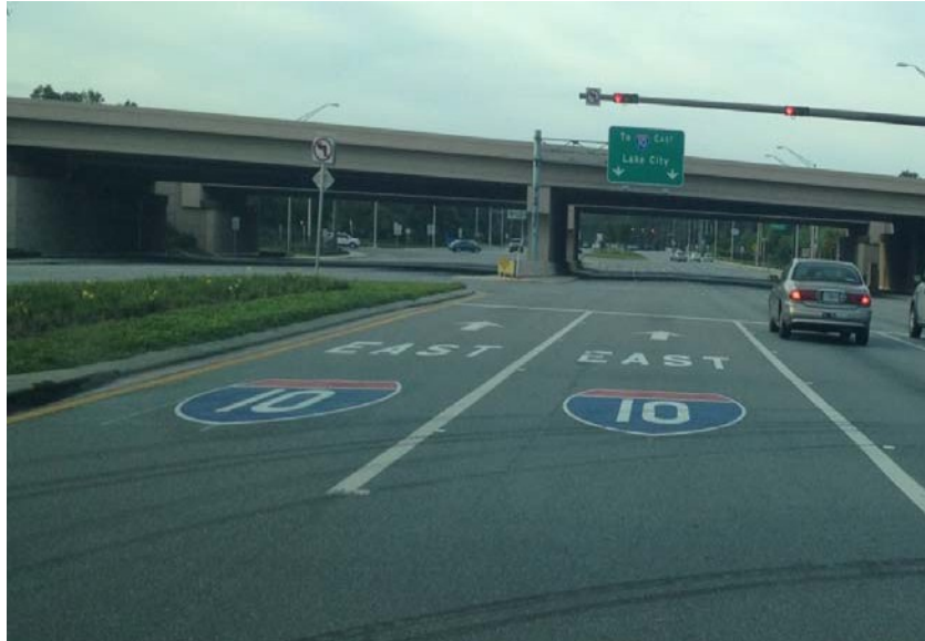
Figure 4.2-7. Pavement Markings for Wrong Way Treatment
