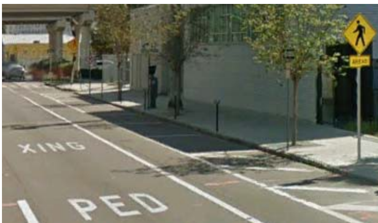
Figure 4.2-1. Pavement Word Markings
