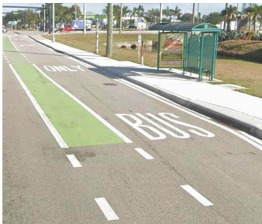
Figure 4.2-1. Pavement Word Markings
