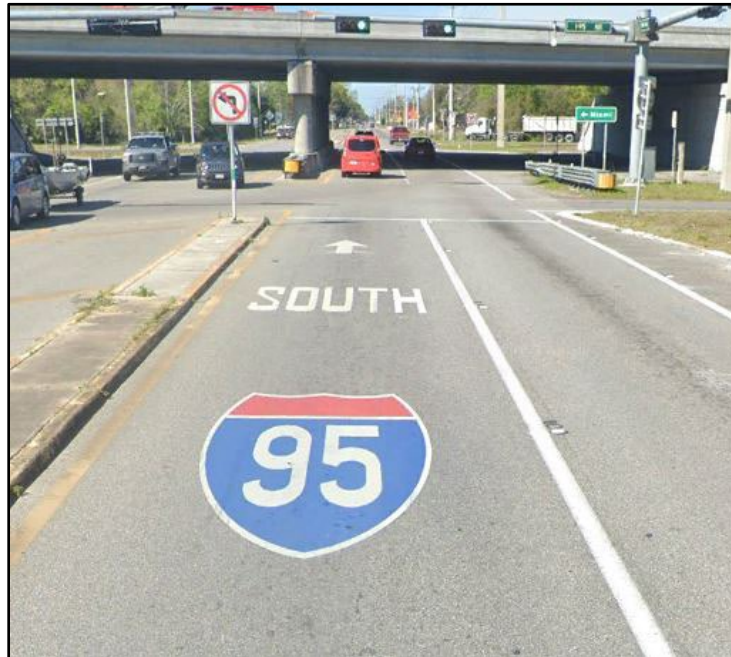
Figure 4.2-6. Pavement Markings for Interchange Access
