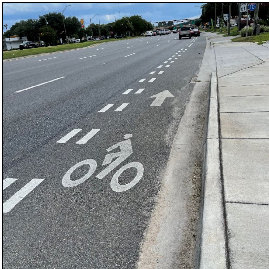
Figure 4.2-2. Pavement Symbol and Arrow Markings
