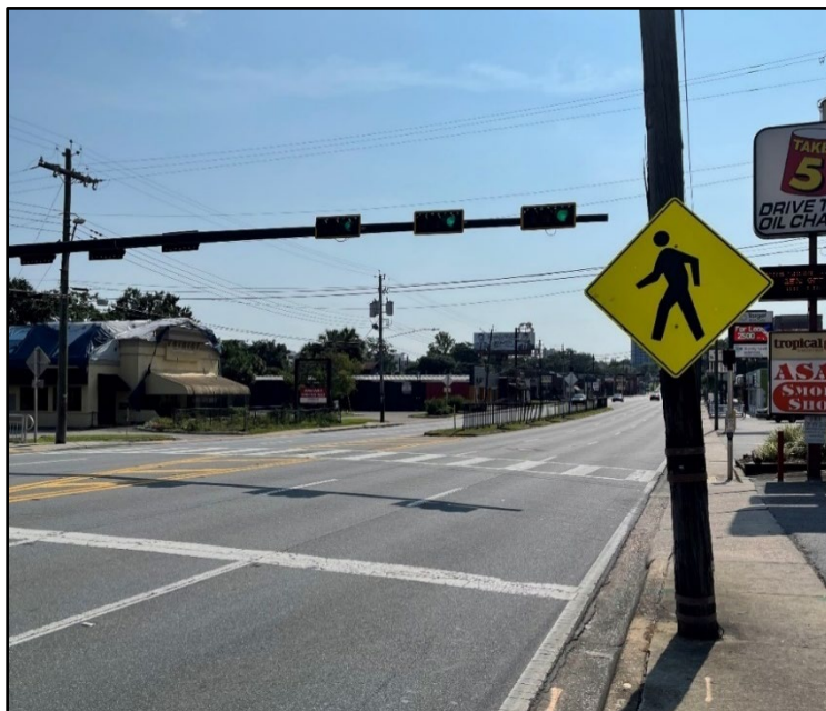
Figure 5.2-10. Midblock Traffic Control Signal
