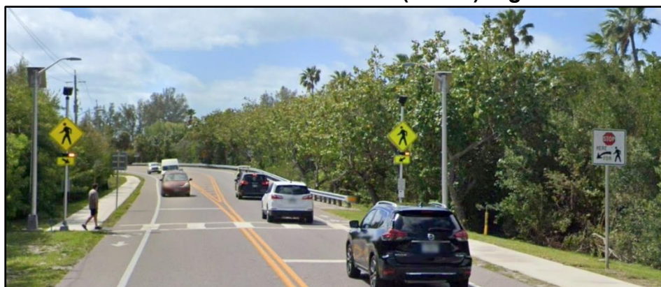
Figure 5.2-4. RRFB with STOP HERE FOR PEDESTRIANS (R1-5b) and PEDESTRIAN CROSSING (W11-2) Signs
