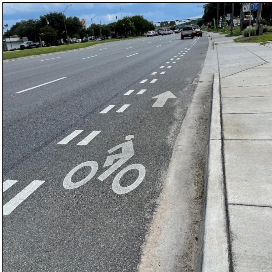
Figure 4.2-2. Pavement Symbol and Arrow Markings
