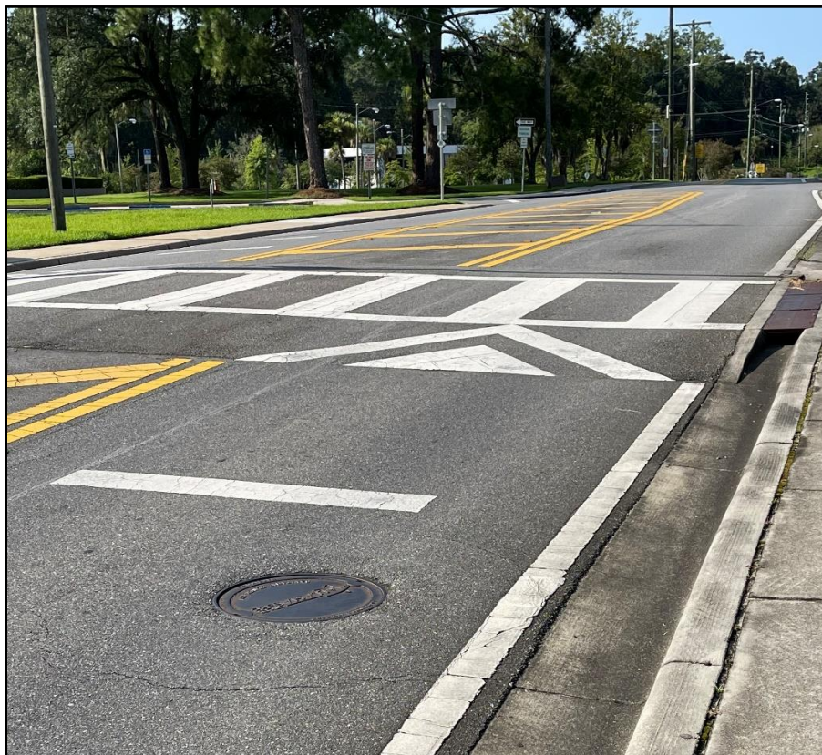
Figure 5.2-11. Raised Crosswalk
