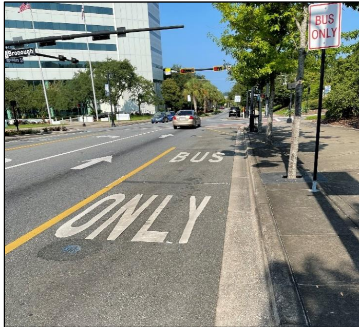
Figure 4.2-1. Pavement Word Markings
