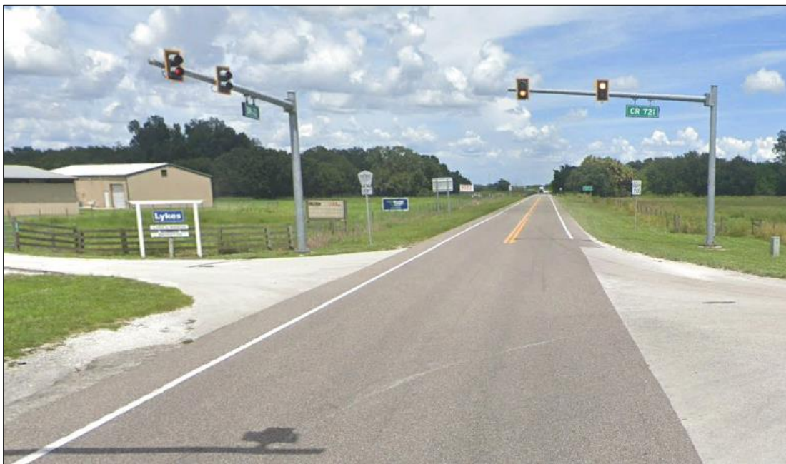
Figure 3.1-1. Intersection Control Beacon
