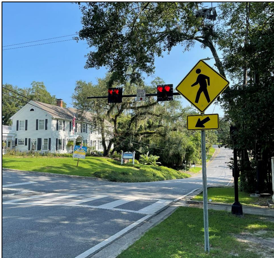
Figure 5.2-9. Pedestrian Hybrid Beacons (PHB)
