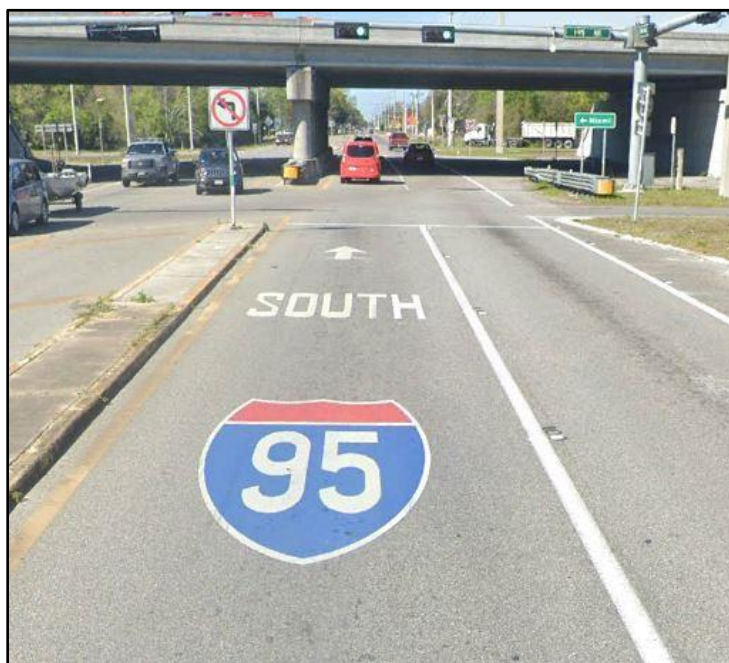
Figure 4.2-6. Pavement Markings for Interchange Access
