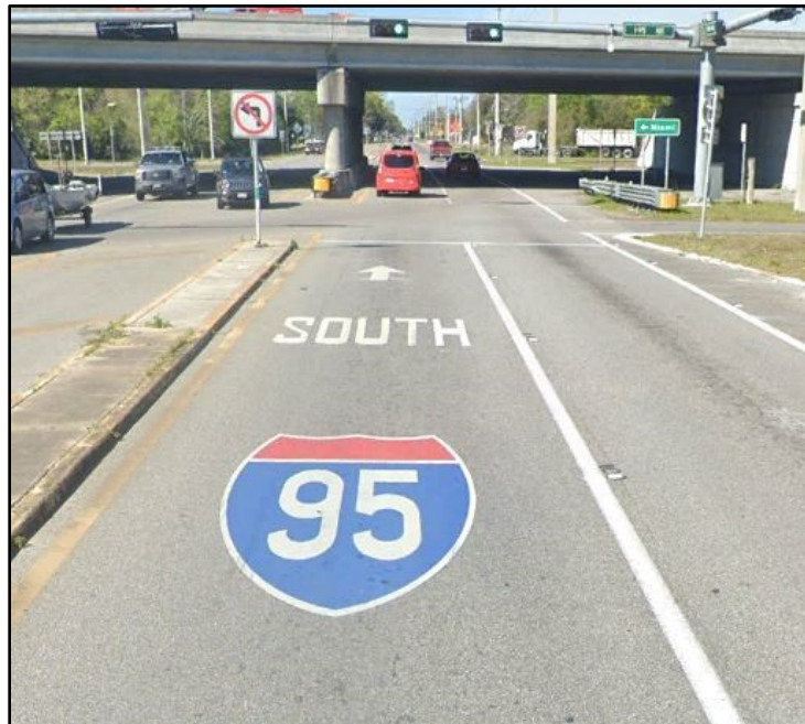
Figure 4.2-6. Pavement Markings for Interchange Access
