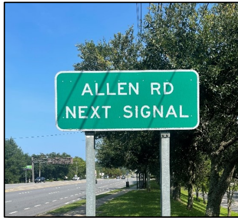
Figure 2.37-1. Advance Street Name Sign at Signalized Locations
