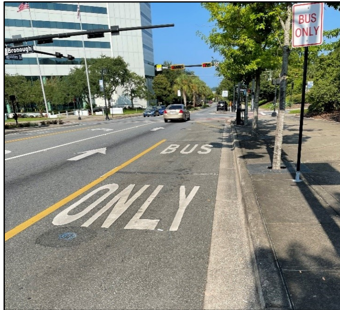
Figure 4.2-1. Pavement Word Markings
