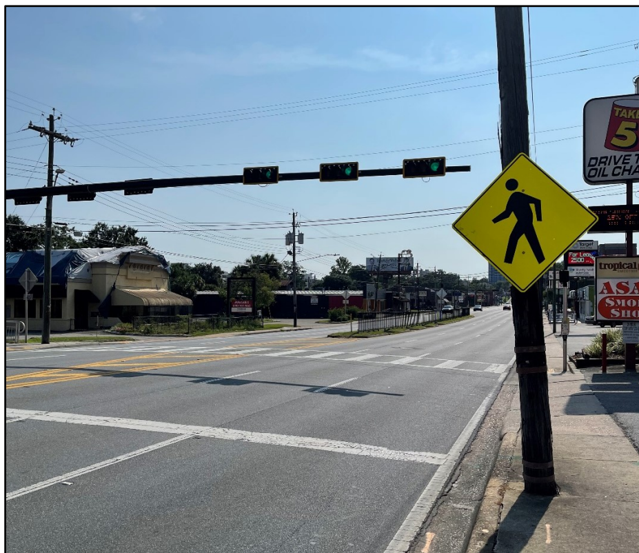
Figure 5.2-10. Midblock Traffic Control Signal
