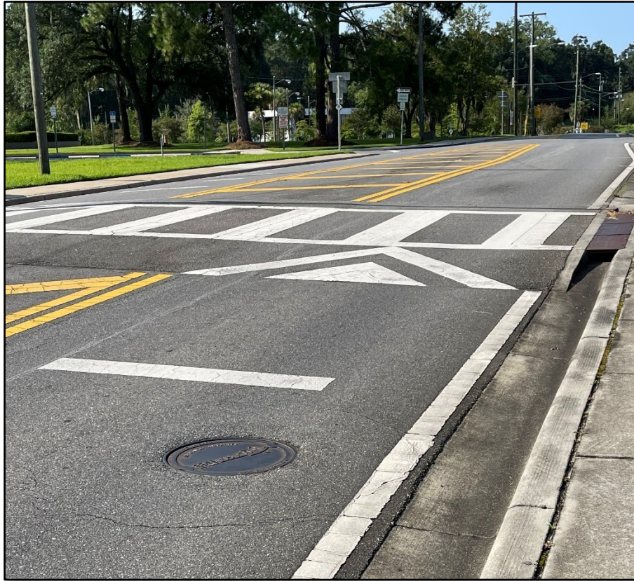
Figure 5.2-11. Raised Pedestrian Crosswalk
