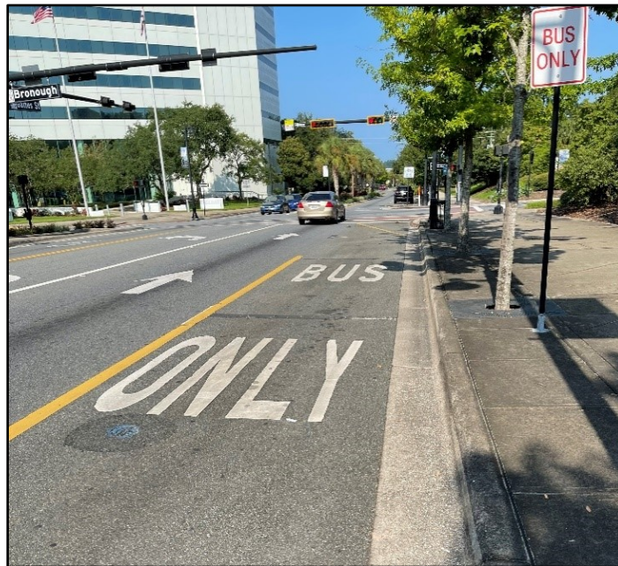
Figure 4.2-1. Pavement Word Markings
