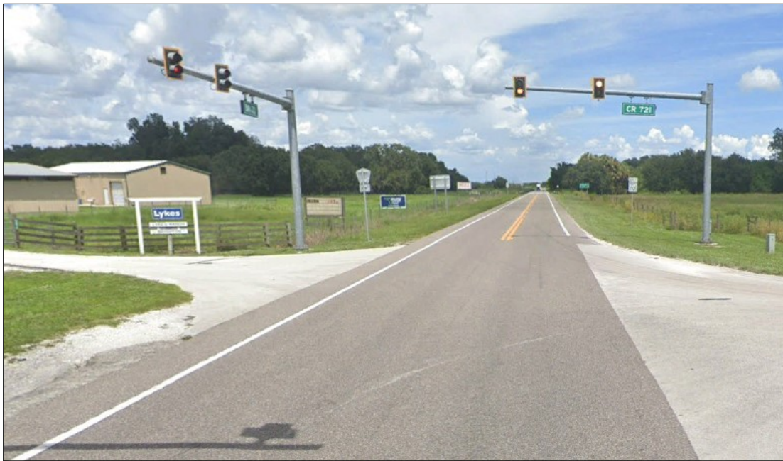
Figure 3.1-1. Intersection Control Beacon
