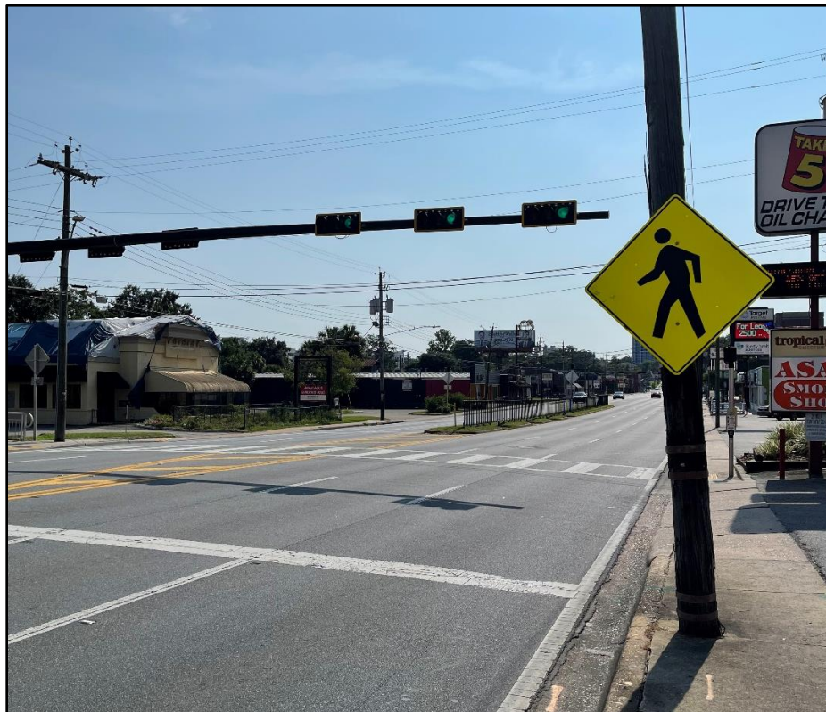
Figure 5.2-10. Midblock Traffic Control Signal
