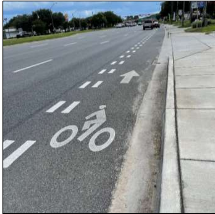
Figure 4.2-2. Pavement Symbol and Arrow Markings
