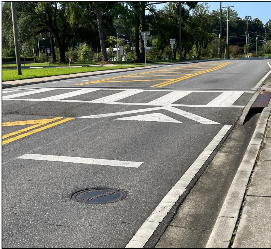
Figure 5.2-11. Raised Pedestrian Crosswalk
