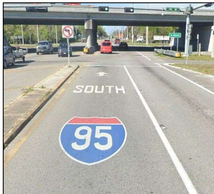
Figure 4.2-7. Pavement Markings for Wrong Way Treatment
