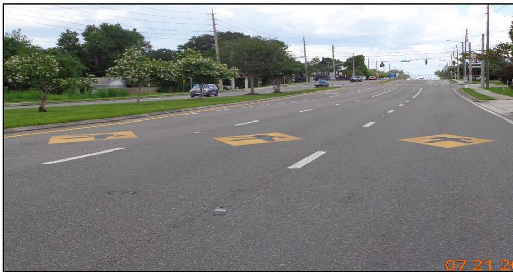
**Figure 5.2-4. PEDESTRIAN and BICYCLE CROSSING WARNING Signs Pavement Marking Details**
