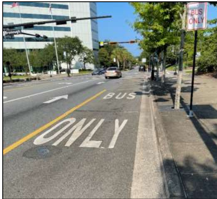
Figure 4.2-1. Pavement Word Markings
