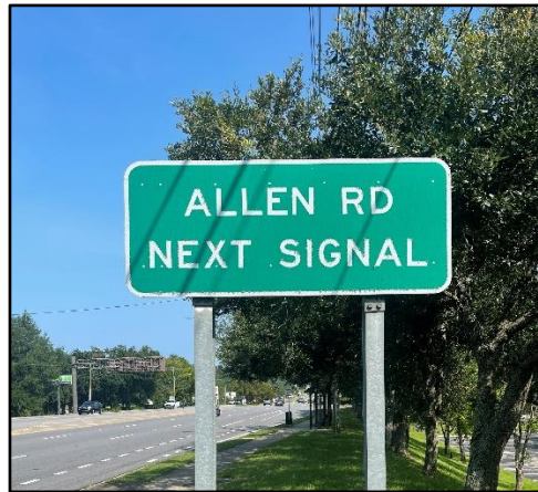
Figure 2.37-1. Advance Street Name Sign at Signalized Locations
