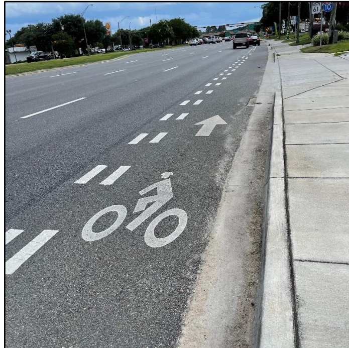
Figure 4.2-2. Pavement Symbol and Arrow Markings
