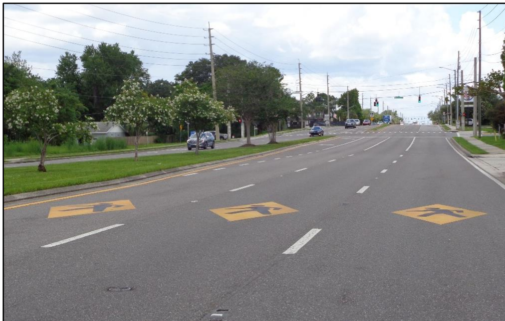
Figure 5.2-3. PEDESTRIAN CROSSING WARNING Sign (W11-2) Pavement Marking
