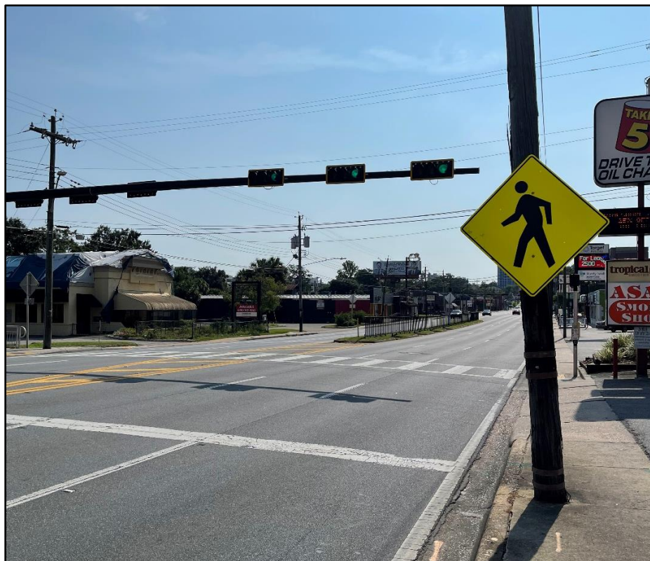
Figure 5.2-10. Midblock Traffic Control Signal
