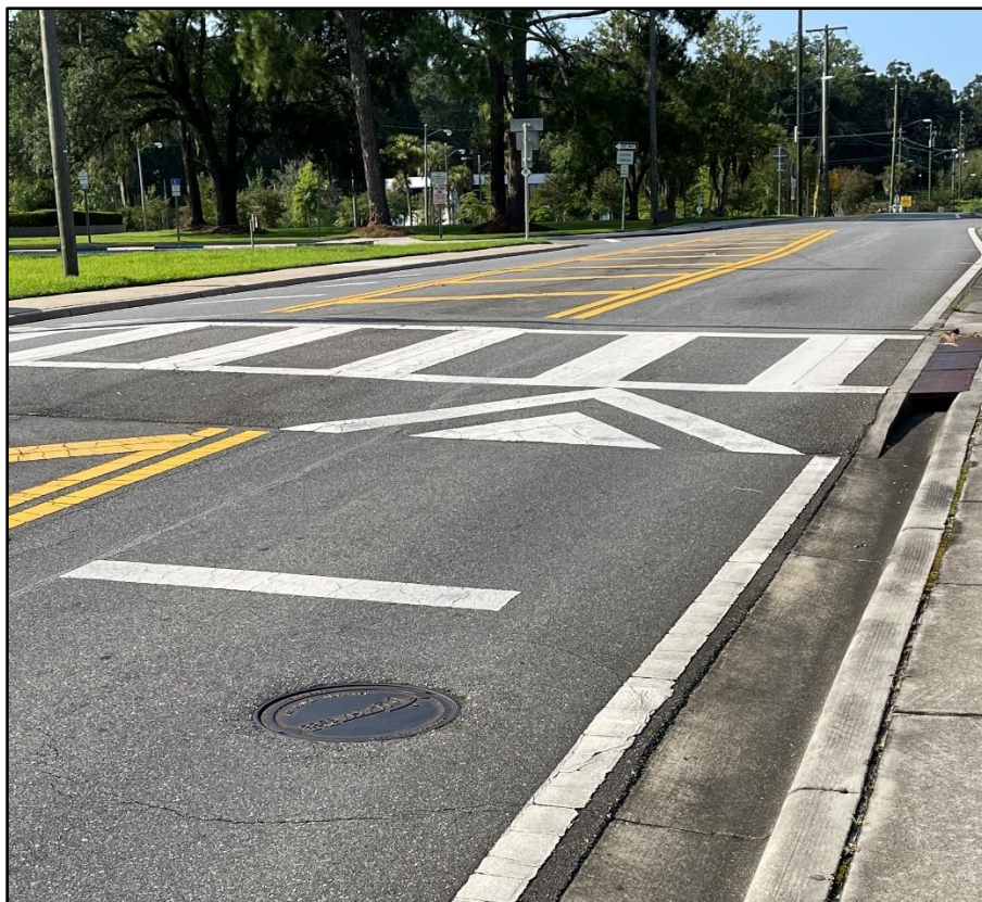
Figure 5.2-11. Raised Pedestrian Crosswalk
