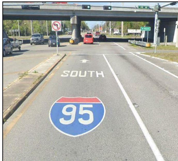
Figure 4.2-7. Pavement Markings for Wrong Way Treatment
