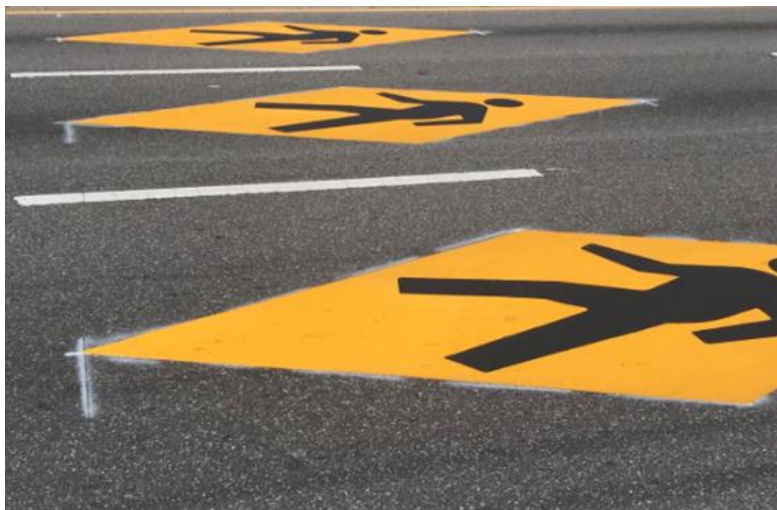
Figure 5.2-3. Pavement W11-2 Marking
