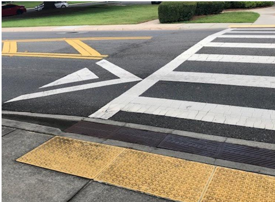
Figure 5.2-9. Raised Pedestrian Crosswalk
