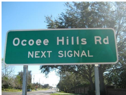
Figure 2.37-1. Advance Street Name Sign at Signalized Locations
