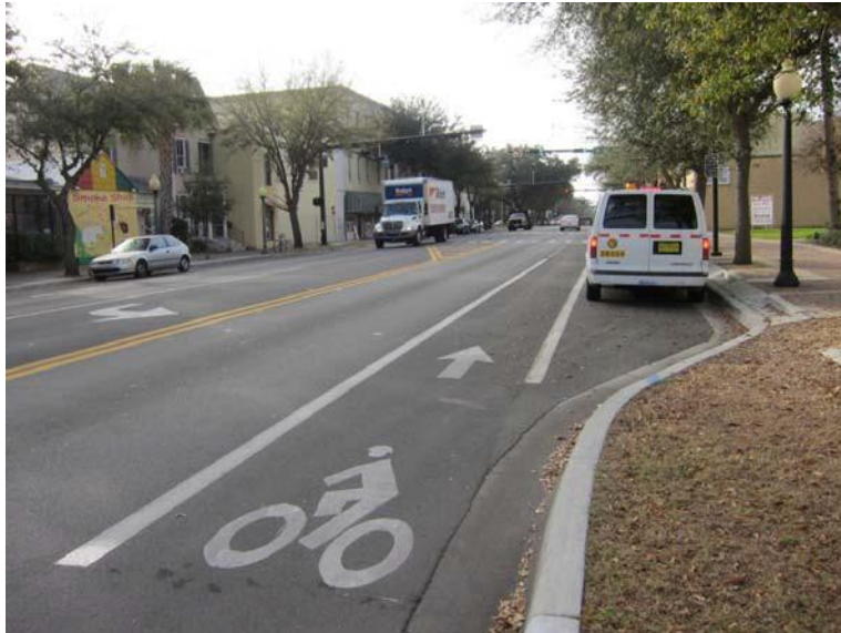
Figure 4.2-2. Pavement Symbol and Arrow Markings
