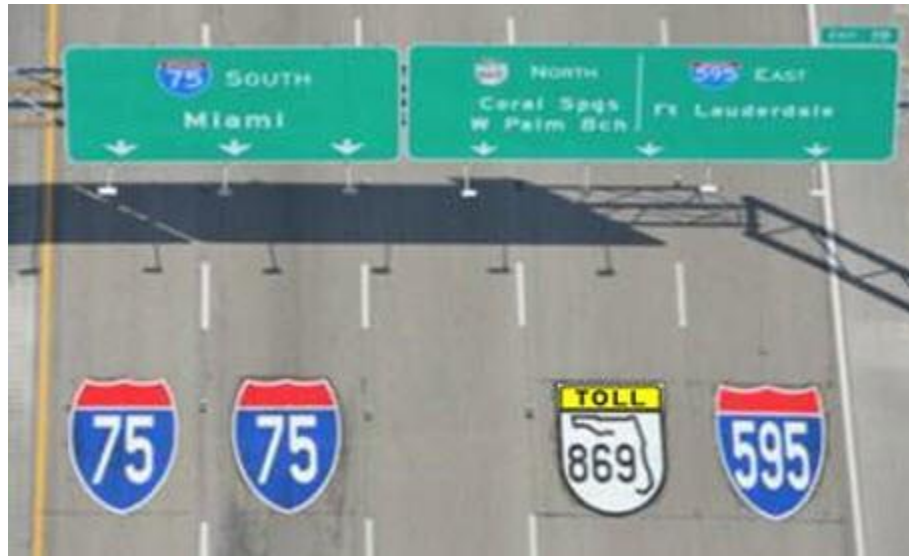
Figure 4.2-3. Route Shield Pavement Markings
