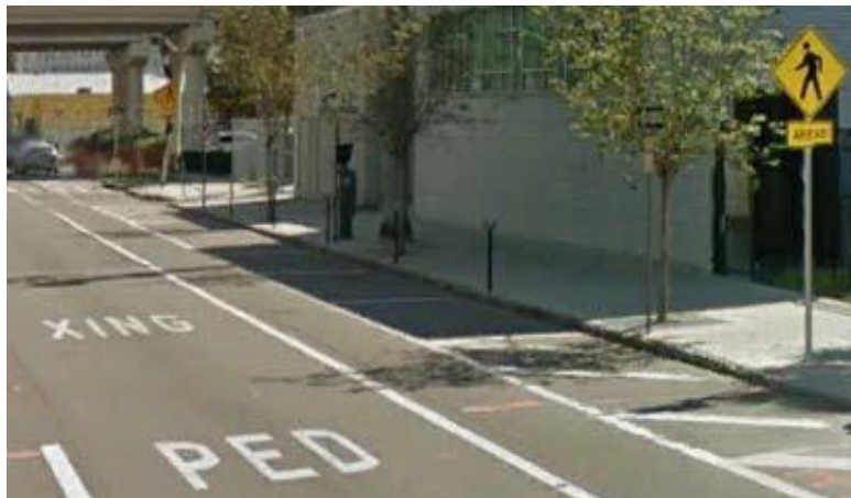
Figure 4.2-1. Pavement Word Markings
