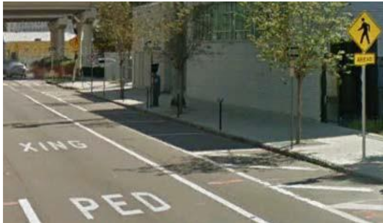
Figure 4.2-1. Pavement Word Markings
