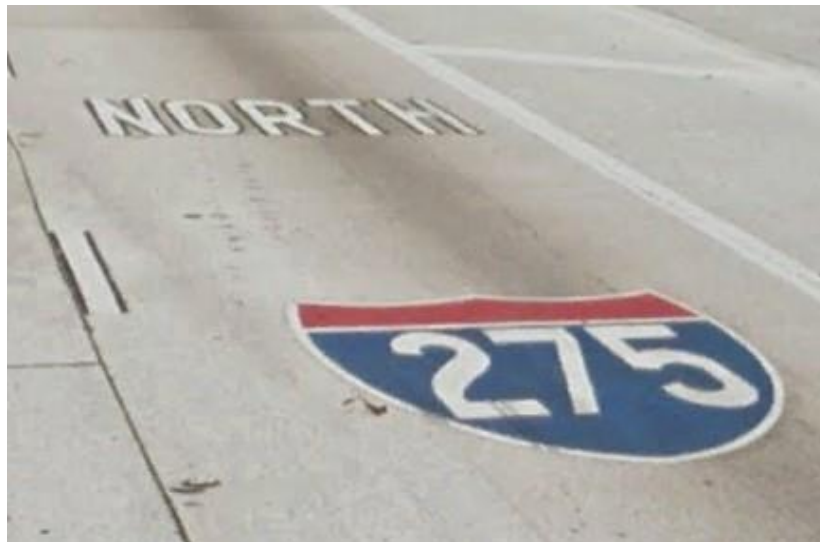
Figure 4.2-4. Cardinal Direction Markings
