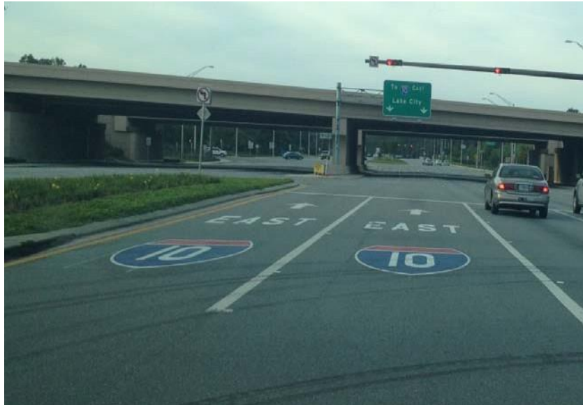
Figure 4.2-7. Pavement Markings for Wrong Way Treatment
