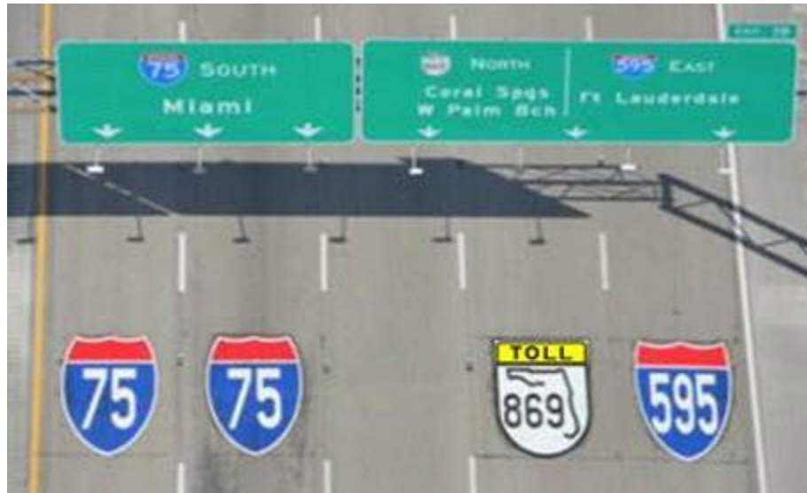
Figure 4.2-3. Route Shield Pavement Markings
