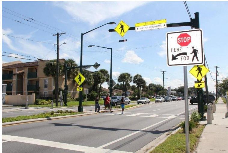
Figure 3.8-4. Rectangular Rapid Flashing Beacons
