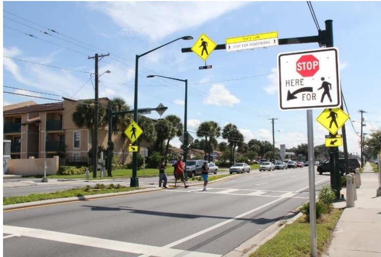
Figure 3.8-4. Rectangular Rapid Flashing Beacons
