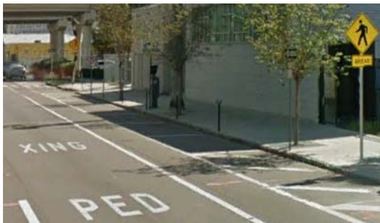
Figure 4.2-1. Pavement Word Markings
