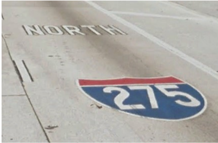
Figure 4.2-4. Cardinal Direction Markings
