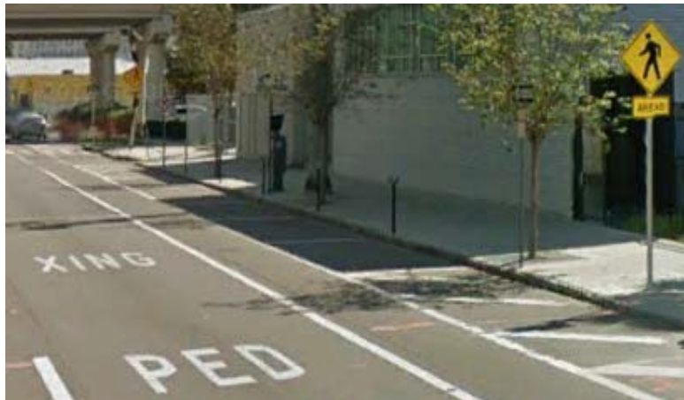
Figure 4.2-1. Pavement Word Markings
