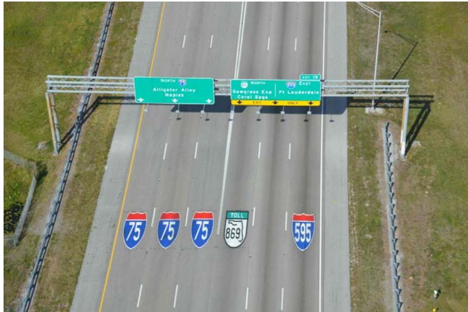
Figure 4.2-3. Route Shield Pavement Markings
