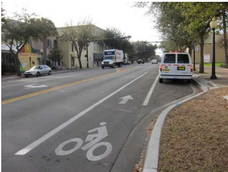
Figure 4.2-2. Pavement Symbol and Arrow Markings
