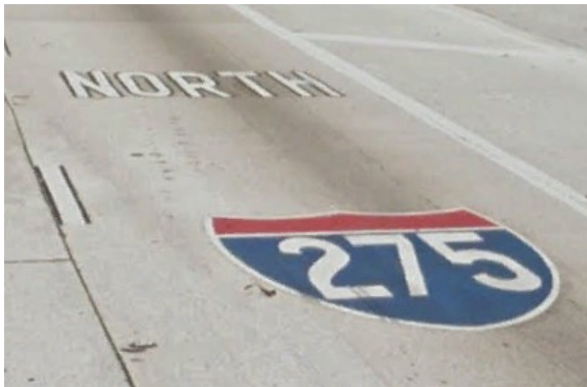
Figure 4.2-4. Cardinal Direction Markings
