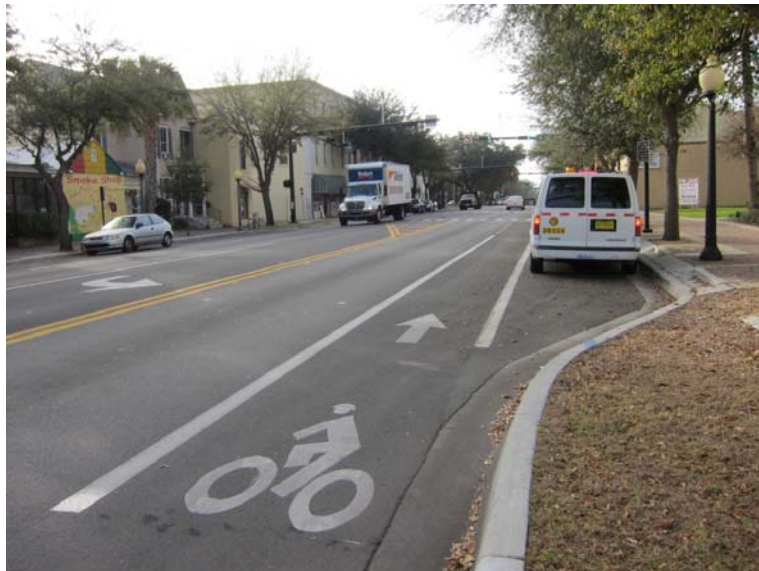
Figure 4.2-2. Pavement Symbol and Arrow Markings
