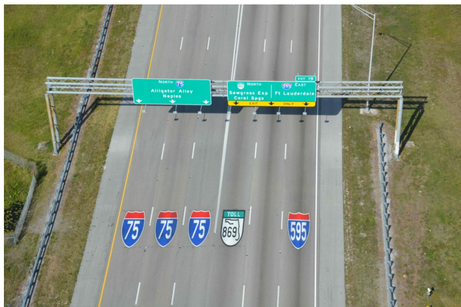
Figure 4.2-3. Route Shield Pavement Markings
