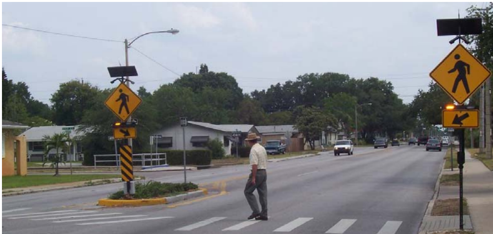
Figure 3.8.3. Rectangular Rapid Flashing Beacons
