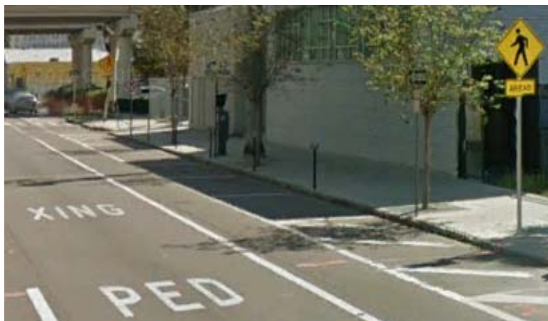
Figure 4.2-1. Pavement Word Markings
