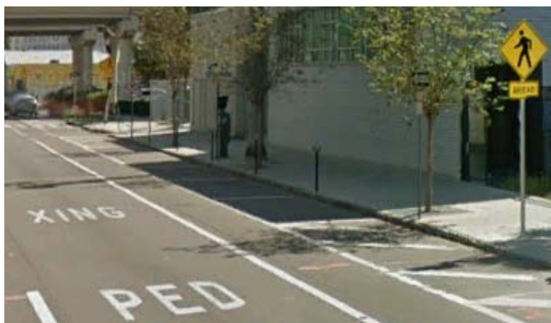
Figure 4.2-1. Pavement Word Markings
