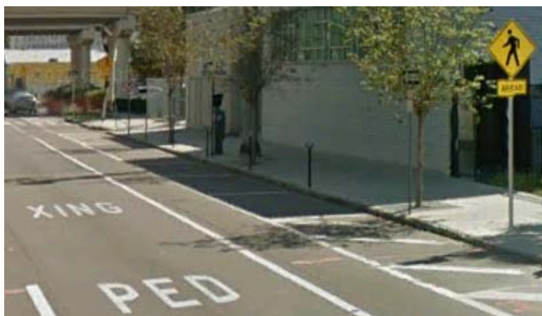
Figure 4.2-1. Pavement Word Markings
