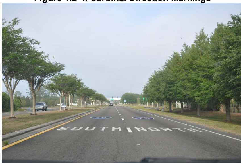
Figure 4.2-4. Cardinal Direction Markings
