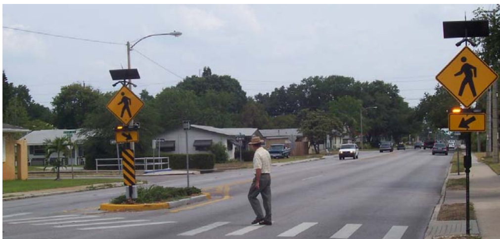
Figure 3.8.3. Rectangular Rapid Flashing Beacons
