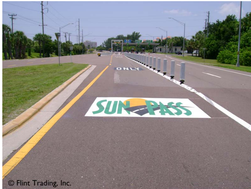
Figure 4.2-5. Expressway Lane Use Message
