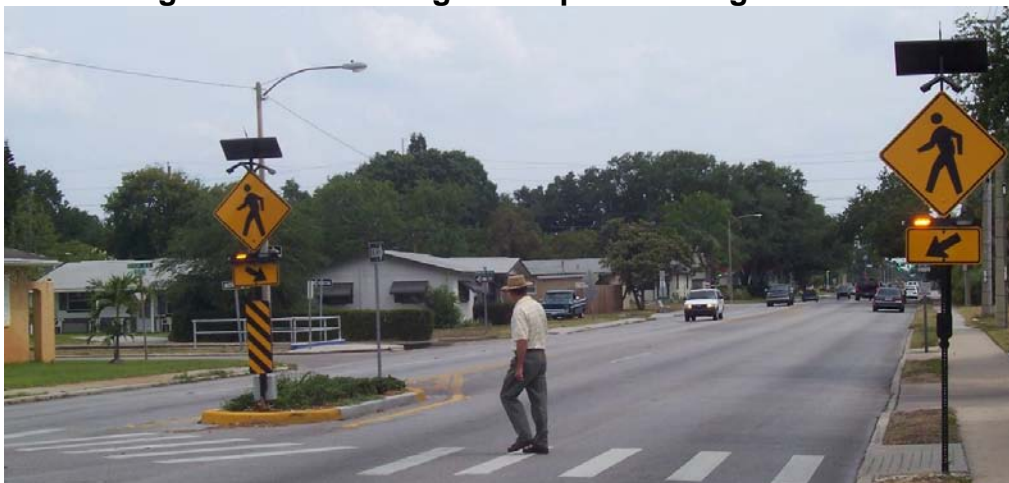
Figure 3.8.3. Rectangular Rapid Flashing Beacons
