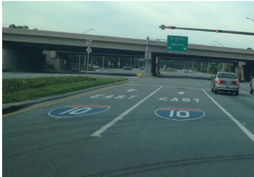
Figure 4.2-7. Pavement Markings for Wrong Way Treatment
