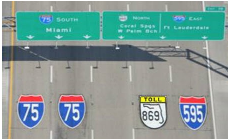
Figure 4.2-3. Route Shield Pavement Markings
