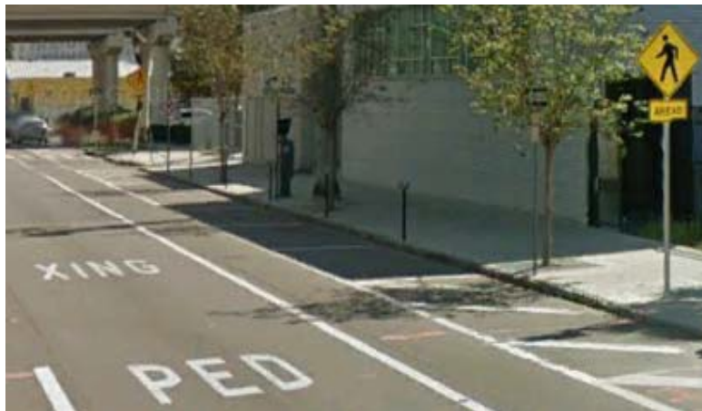
Figure 4.2-1. Pavement Word Markings
