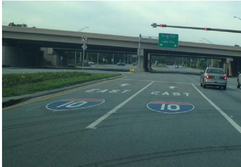
Figure 4.2-7. Pavement Markings for Wrong Way Treatment
