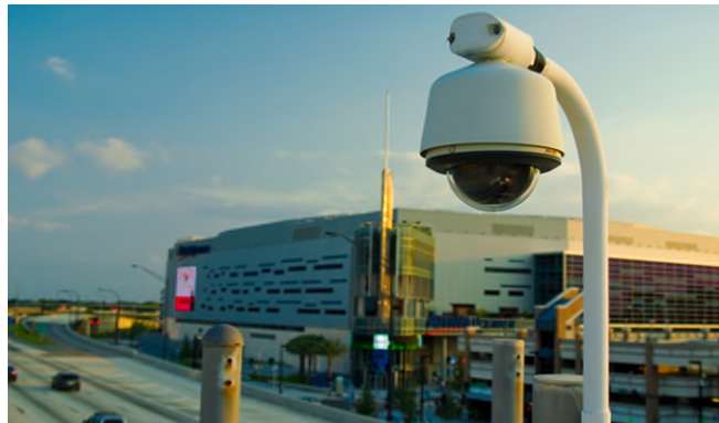
Figure 6: CCTV Camera on I-4 in Orlando
