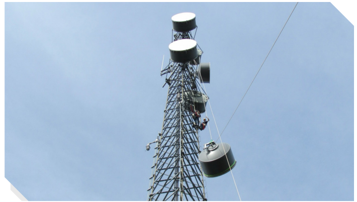
Figure 2 - Installation of new High Performance Microwave Antenna
