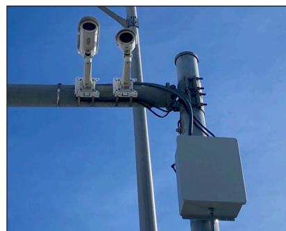
Figure 5: Welch Causeway FLIR
