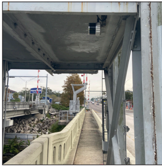
Figure 3: Hillsborough River Bridge LiDAR Sensor
