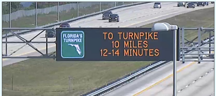
Travel time message on a graphic-enabled sign on FTE's Sawgrass Expressway (SR 869) in Broward County.
