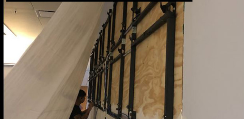
July 17, supports for the video wall
