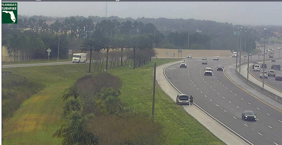
Disabled vehicles are a traffic hazard on their own, but when you add a pedestrian standing alongside their vehicle on a high-speed roadway, the risk of a life-threatening event increases exponentially.
