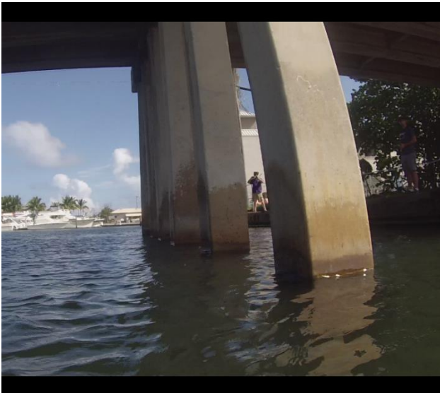
Figure 73: Above water and underwater images of the southern row of pilings showing multiple pilings imaged at the same time. In these images, the distance from the pilings is a bit further than in the previous images. One can see that the sonar images are taken at somewhat of an oblique angle and the condition of the pilings is not as clear as it is in the previous images. However, some of the streambed features are more easily visible from this vantage point.
