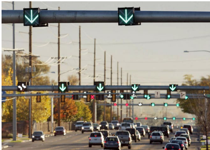
Figure 2.8 - Flexible-Lane Signalization Infrastructure: Despite their efficiency, flexible lane systems today require cumbersome infrastructure to keep roadways safe. AV systems will allow for the benefits of directionally flexible roads without the expensive and unsightly infrastructure investments.
