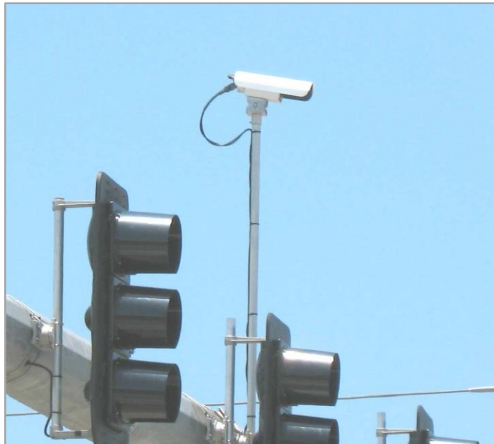
Figure 10: Camera Extension for Additional Mounting Height
